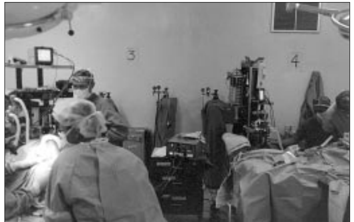
Figure 3. Two anesthesia machines supplied by one nitrous oxide tank.
